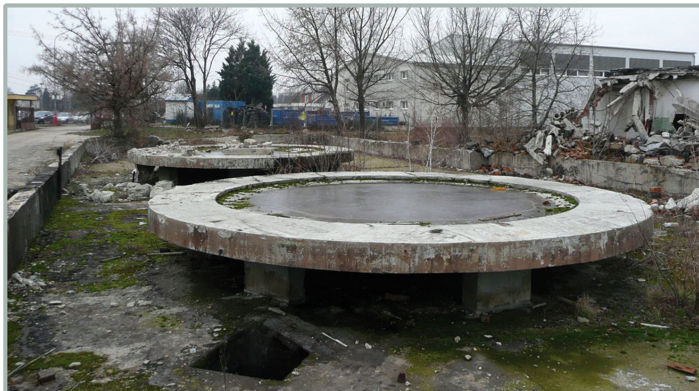
Nitra - Chrenová, mazutová kotolňa (probable contaminated site)
